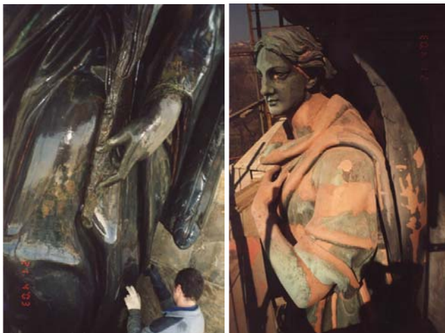
Fig. 9. Restoration of the lost copper coating at the antique sculptures of Isaac Cathedral in Saint-Petersburg.
