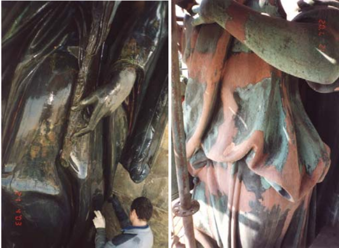
Figure 13: Restoration of the lost copper coating at the antique sculptures of Isaac Cathedral in Saint-Petersburg.
